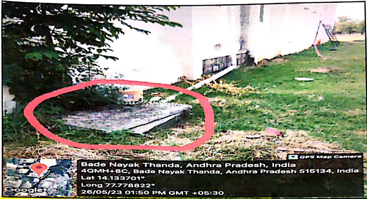
Fig: Rain water harvesting pit of near SSE Power Generator room
