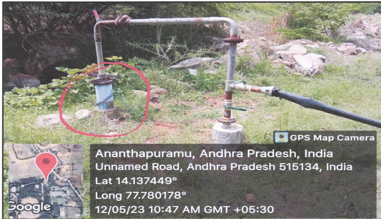
Fig: Borewell point near SSE entrance gate
