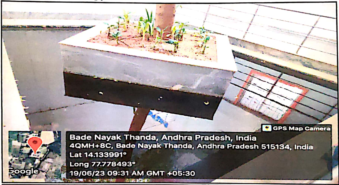
Fig: Rain water storage from SSE first and second floor
