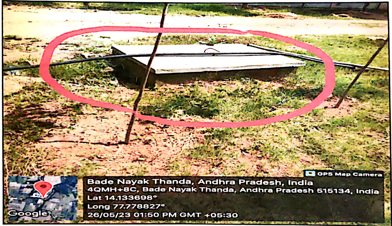
Fig: Rain water harvesting pit of near SSE Power Generator room
