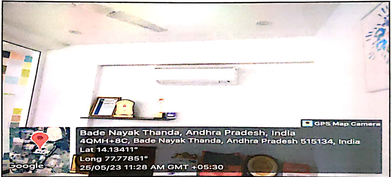
Fig: power efficient electronic devices in SSE staff rooms
