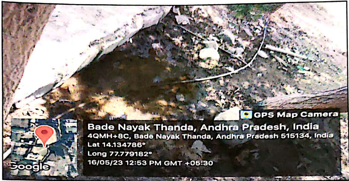
Fig: Rain water harvesting pit at SSE
