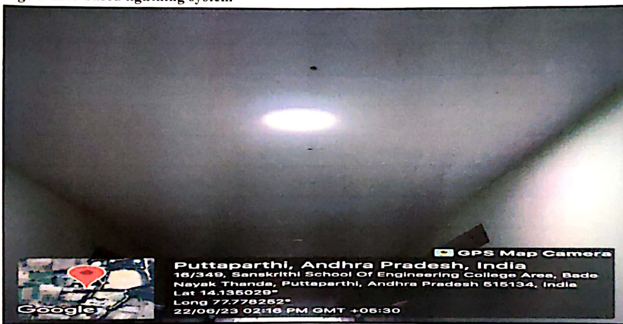
Fig: Sensor based lightning system
