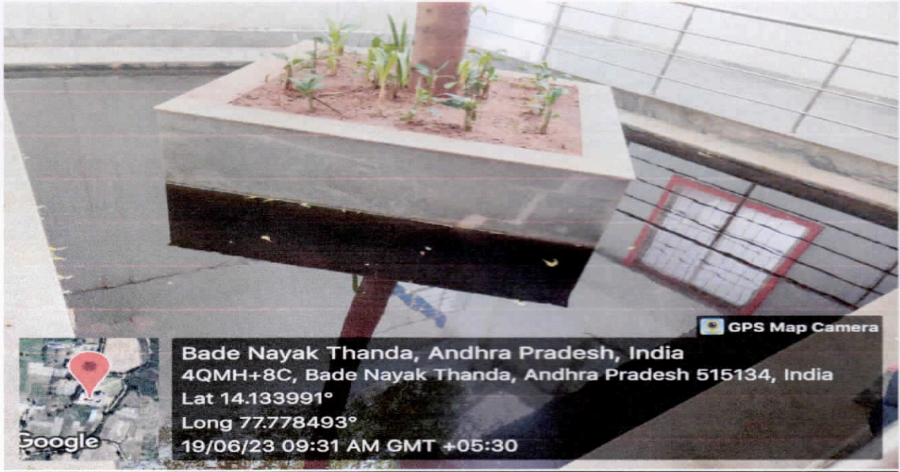
Fig: Rain water storage from SSE first and second floor
