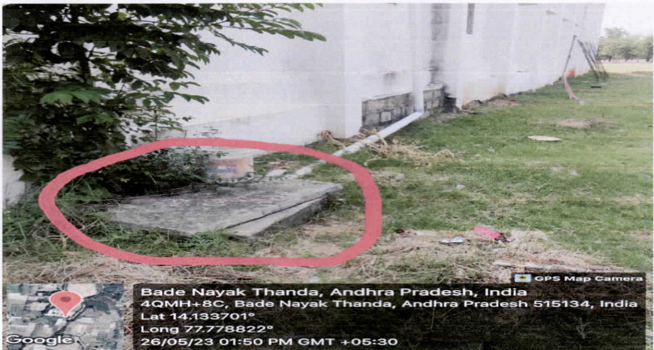
Fig: Rain water harvesting pit backside of Main building
